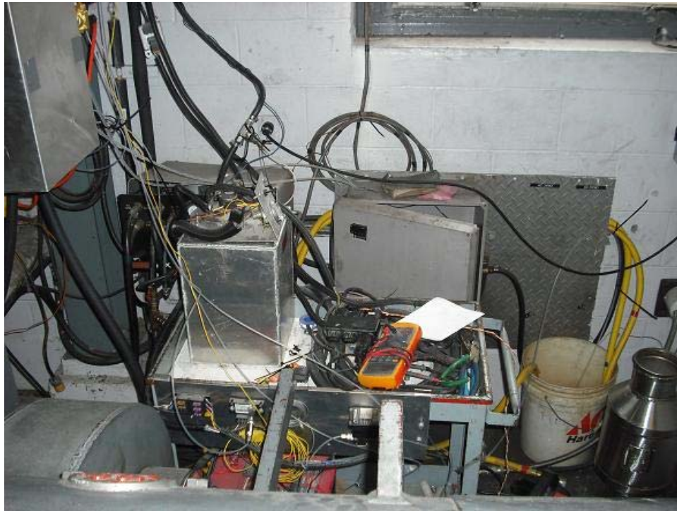
Figure 31. Urea-SCR system instrumentation cart
